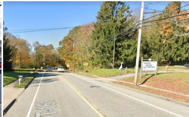
Portion of Route 161 with shoulders on both sides. Source: Google Streetview
