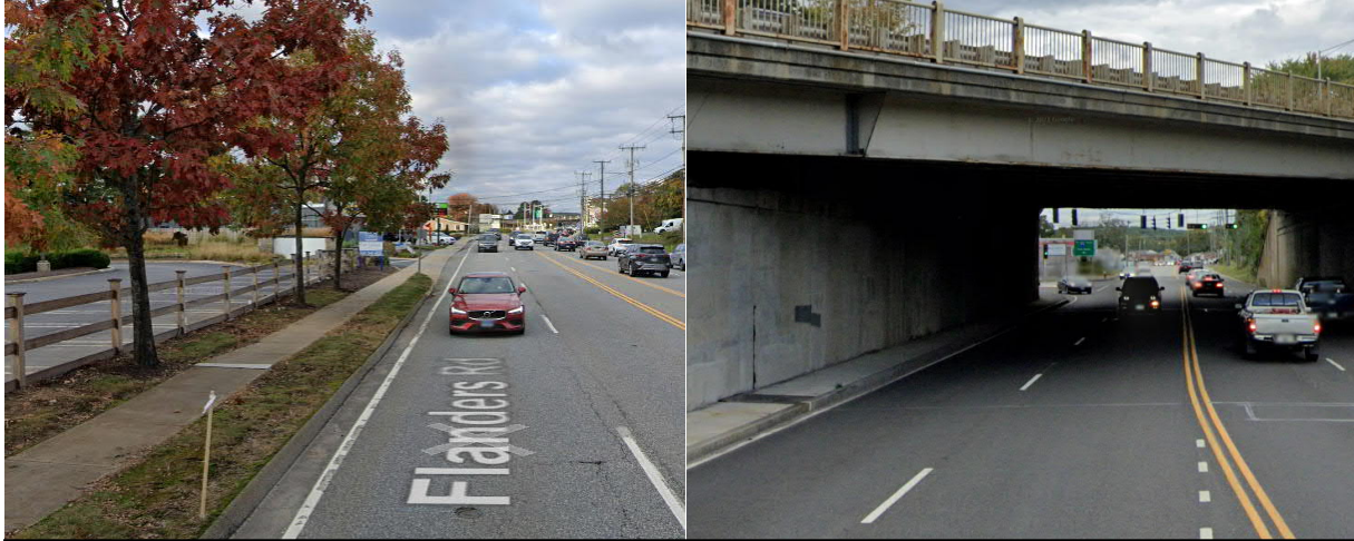
Route 161 by Stop and Shop (Left) with grass buffer and tree. Underpass (Right) with dark narrow sidewalk provided. Source: Google Streetview
